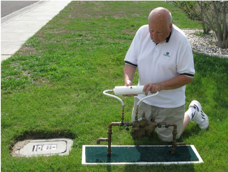
**Method 2** utilizes a refrigerator ice water filter cartridge from Home Depot. The filtering medium is replaced with a toxic granular pesticide or herbicide which then contaminates the drinking water as it flows on into a home, school, commercial building or a government facility to the right.
